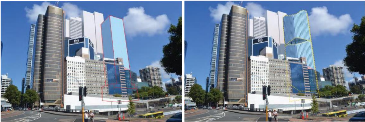
Figure 14: View from Alfred Steet southeast of the site, with the compliant envelope on the left and the proposed building to the right (Ethos Urban).
