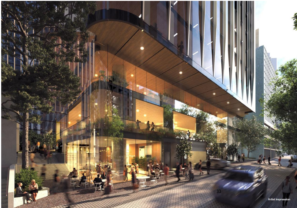
The ground plane from Little Walker Street, the pedestrian link is to the left.
